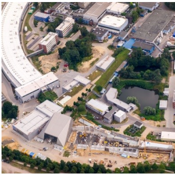
Fig. 1: Aerial View of the entire FLASH facility at DESY including the new tunnel (on the left side) and the new experimental hall (in the lower left corner) in July 2014. The curved PETRA III hall (left) and the construction site of the PETRA extension North (in the lower right corner) are adjacent to the two FLASH experimental halls.
